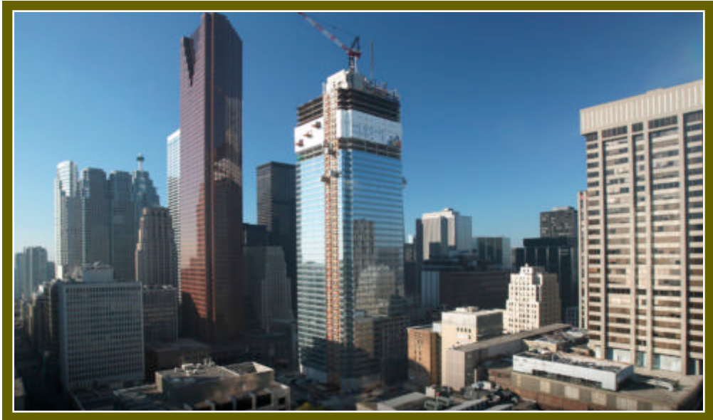
Bay Adelaide Centre, Toronto, under construction
